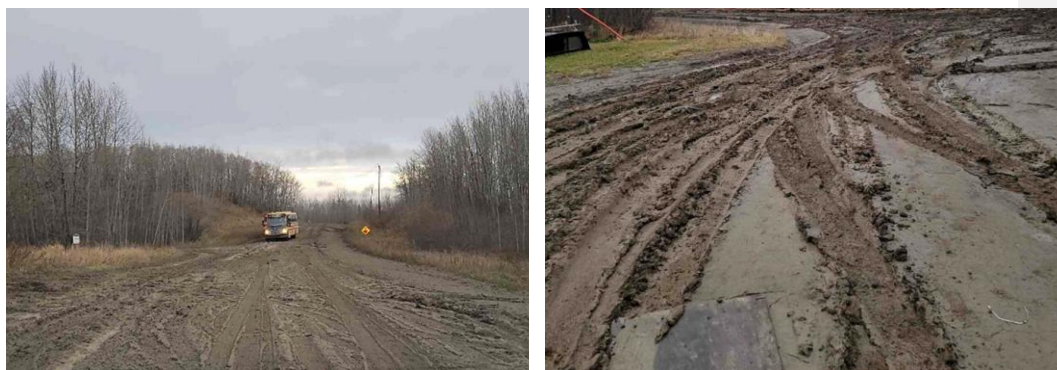
FIGURE 12: ROAD CONDITIONS IN PAUL FIRST NATION, ALBERTA
